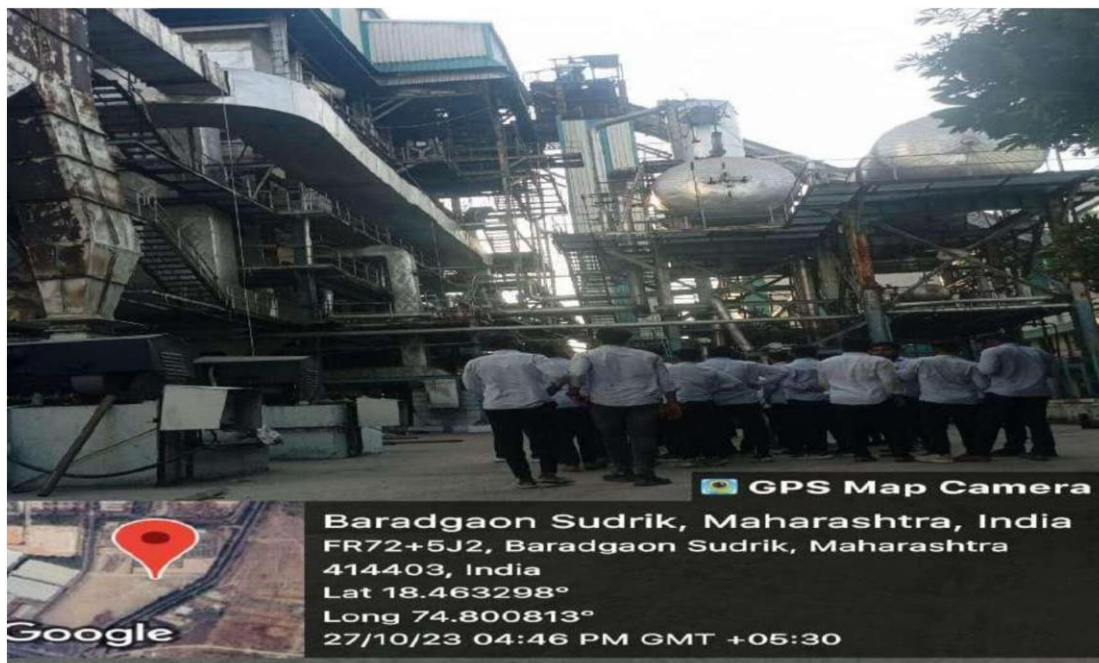
ELECTROSTATIC PRECIPITATOR TO COLLECT THE SUSPENDED PARTICLES GENERATED FROM THE INDUSTRY
