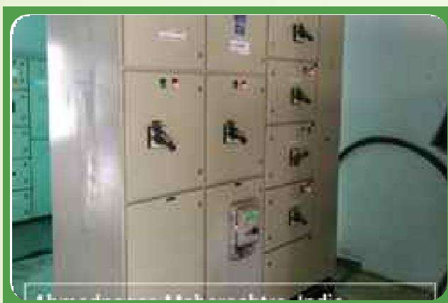
Figure 4 : Meter and inverter panels
