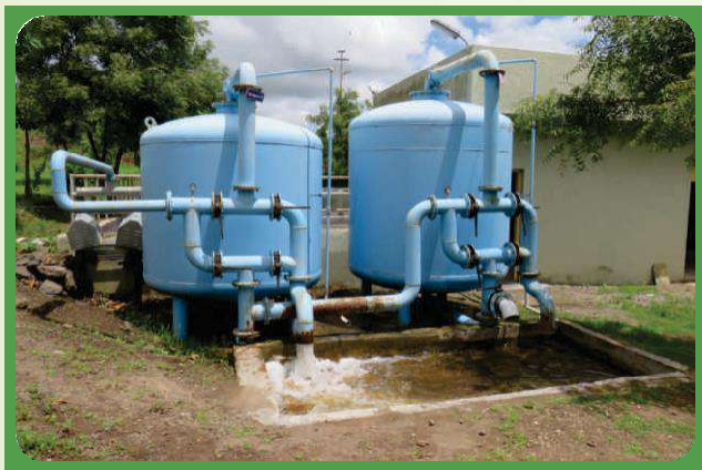
Figure 16 : STP filters and air compressor
