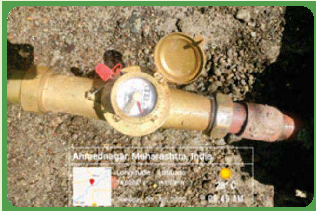
Figure 17 : Water meters installed in campus
