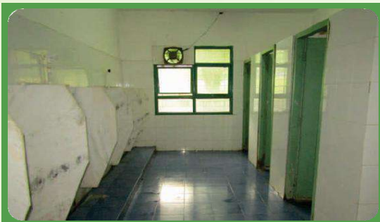
Figure 31 : Exhaust fans in toilet and store
