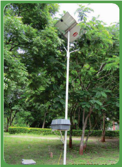
Figure 6 : Solar powered street lights
