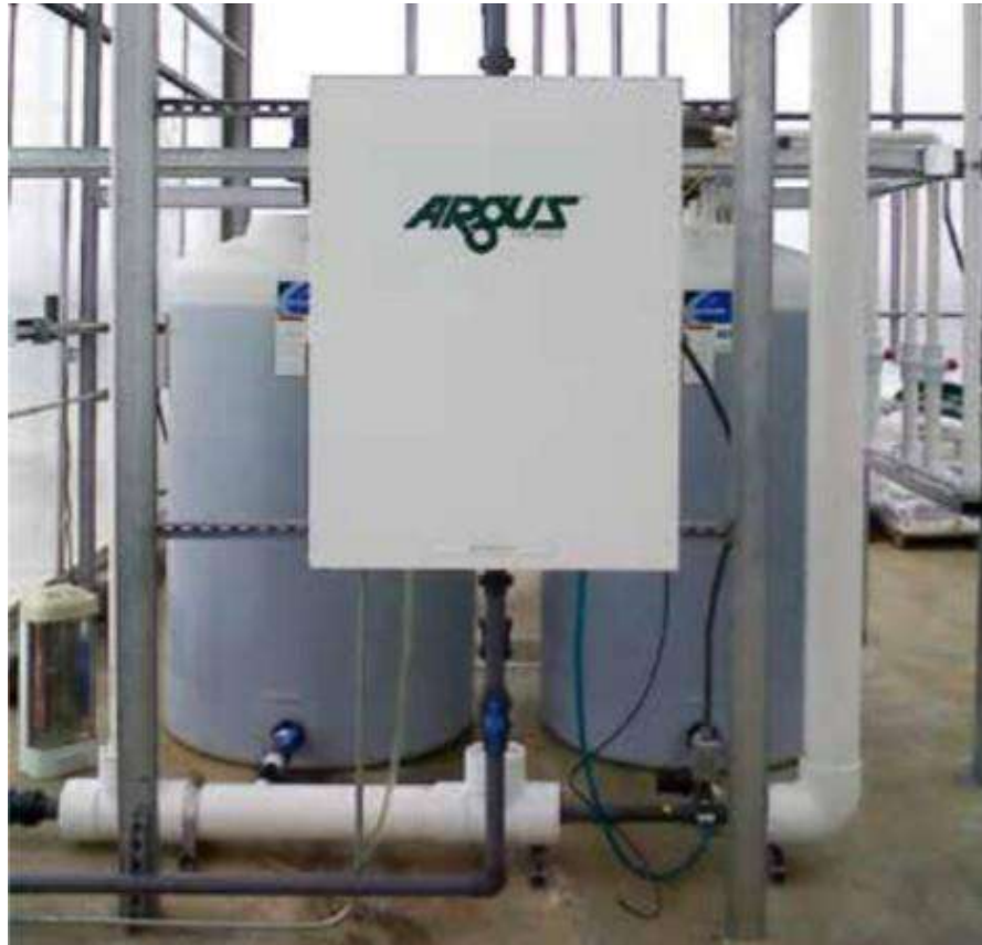
Figure 21: In-Line Injection Dosing System
