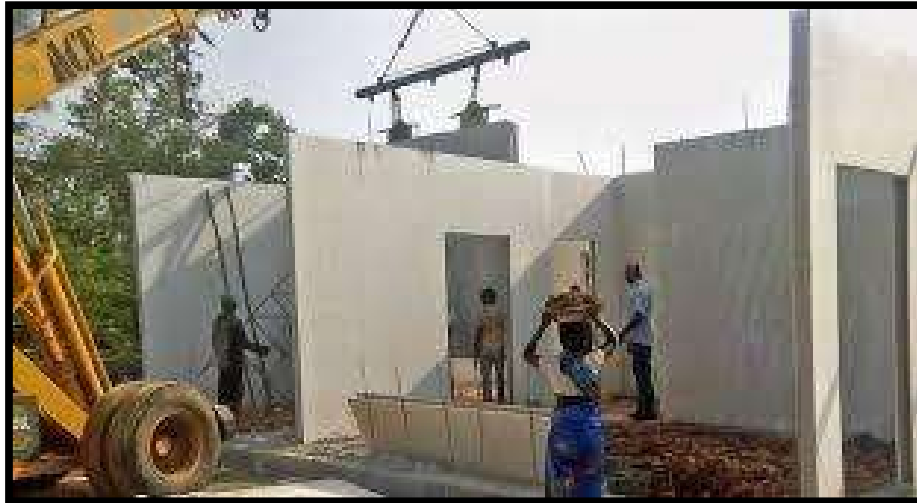
Figure 2. Erection of GFRG Panel
