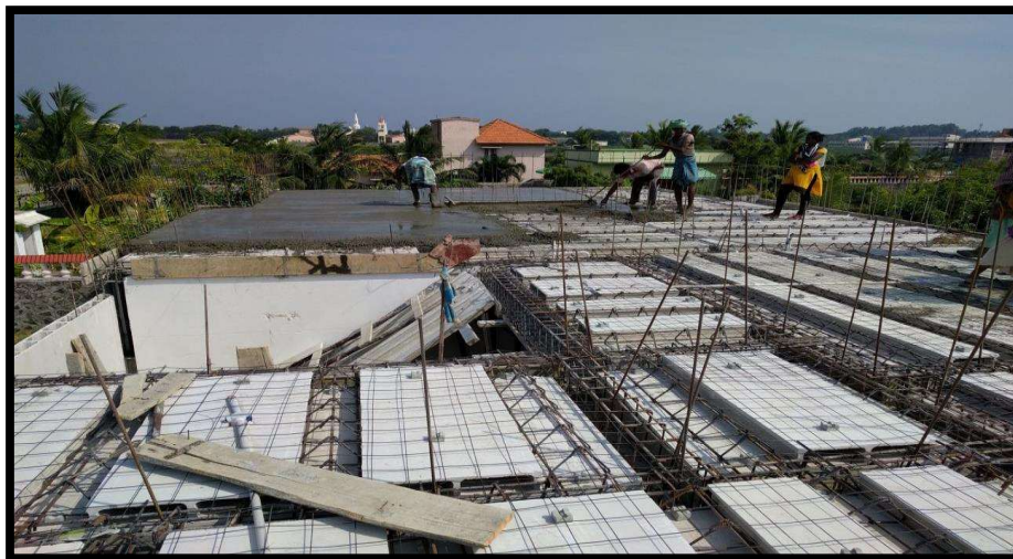
Figure 3. Embedded RCC tie beam
