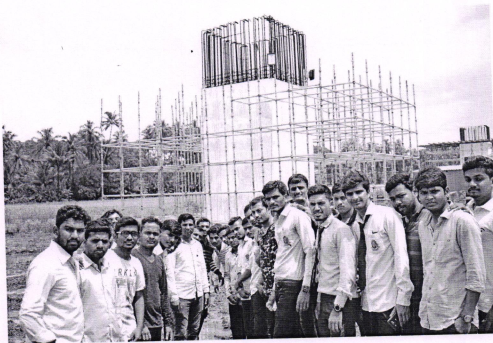
A visit to under construction bridge on Mumbai Goa Highway NH 17
