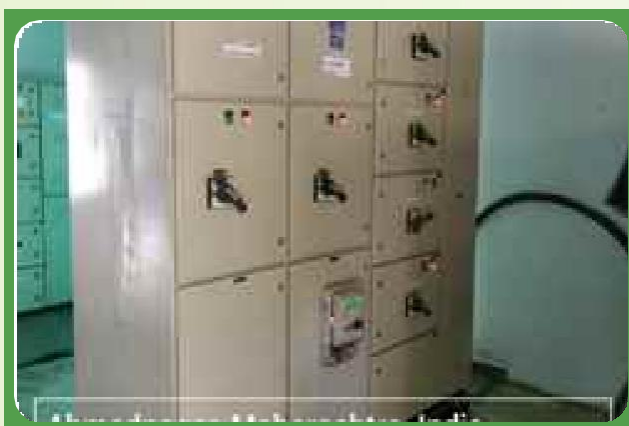
Figure 4 : Meter and inverter panels
