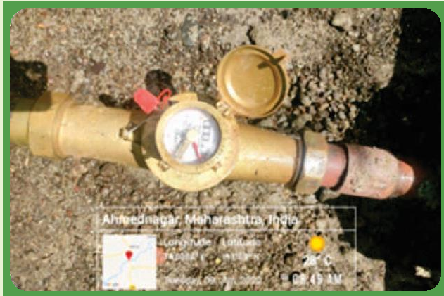
Figure 17 : Water meters installed in campus
