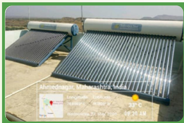
Figure 7 : ETC and FPC solar water heating system
