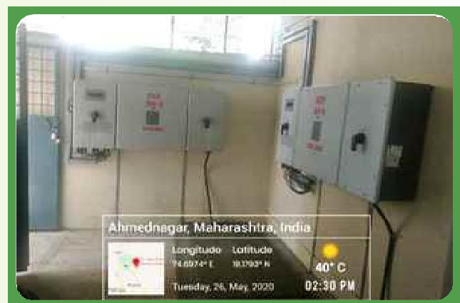
Figure 4 : Meter and inverter panels
