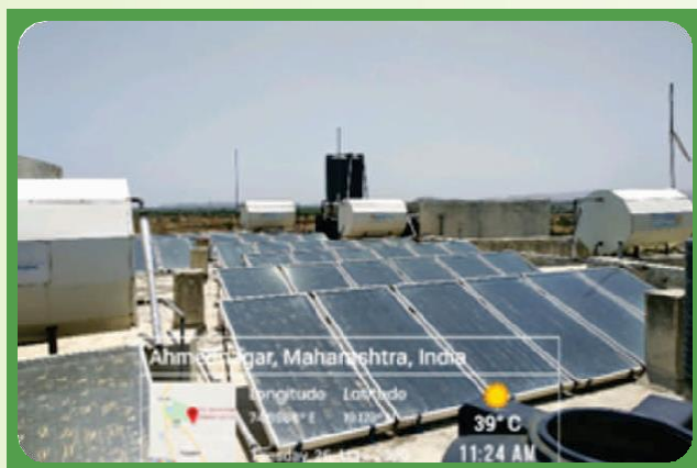
Figure 7 : ETC and FPC solar water heating system
