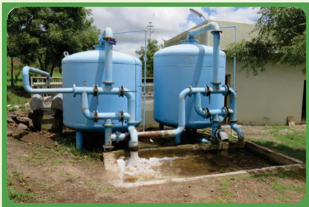
Figure 16 : STP filters and air compressor
